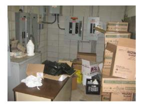
The circuit breakers in the Motor Pool shop of building one are taped open. This is not permitted. The breakers need to be free to trip without tape. Recommendation 3-2016 (I)
